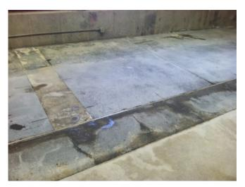
**After:** 1 week after surface was cleaned Cover-Clean HC. No sign of oil "bleed back" Two applications of CoverClean HC were necessary. One at full strength. The second at a 2:1 dilution.
