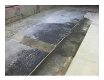
**Before:** Oil stained substrate used to stored construction plant and equipment. Concrete subject to 20 yrs of oil contamination from motor and hydraulic oil.
